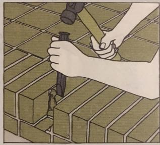
With a hammer and cold chisel, chip out the damaged brick. Take care not to disturb adjacent bricks
